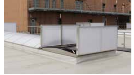
NSHEV type PHOENIX at the end of a EUROLIGHT MKIII continuous rooflight
